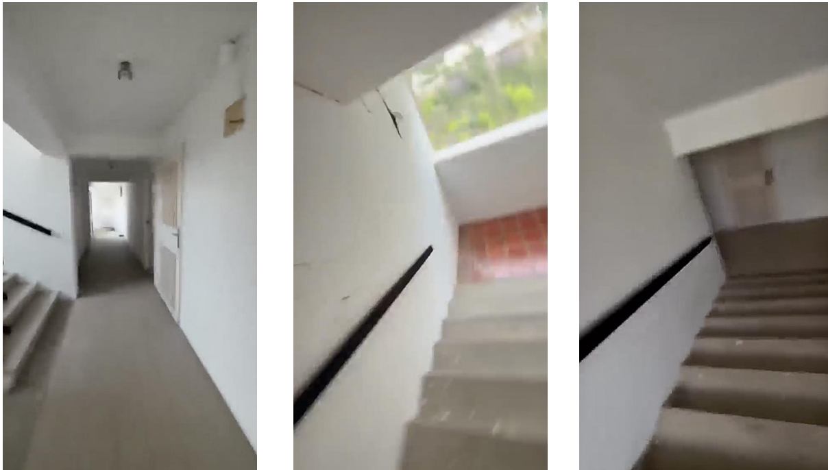
Figure 1: Representative condition of upper stories showing intact finishes, minor hairline cracking, and lack of debris accumulation.
